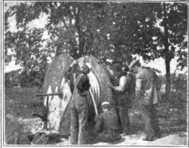
Fig. 23.—Feeding Cable Into Vault.
